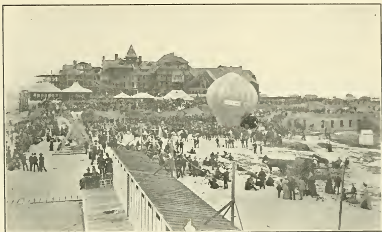
HOTEL DEL CORONADO DURING CONSTRUCTION
